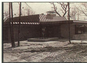
1965 Construction begins on the Student Center in Pasadena, a gymnasium in England and a dormitory complex in Big Sandy.
